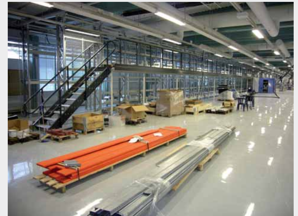
AWA's reel handling system getting its shape in January 2008
